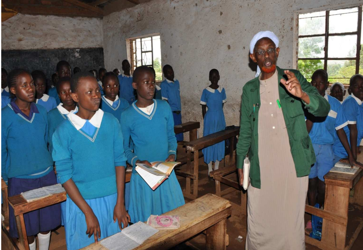
NACCSC Member, Mr Hassan Sheikh Ali addressing the pupils: The classroom was poorly constructed
