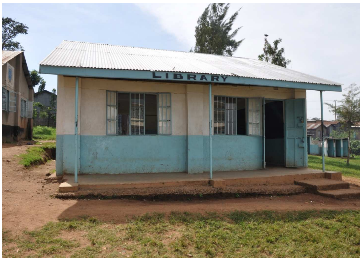
A Library project at Bondeni Primary School
