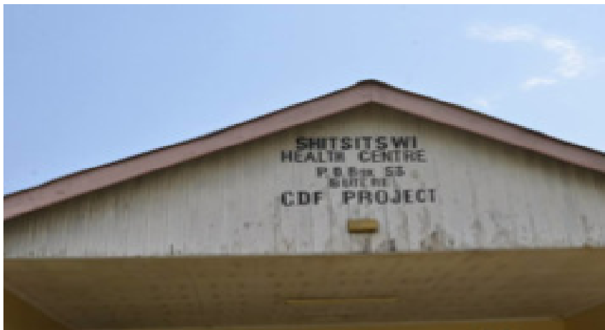
Shitsitwi Health Centre in Butere SubCounty was funded by The Constituency Development Fund at a cost of Ksh.5.32 Million
