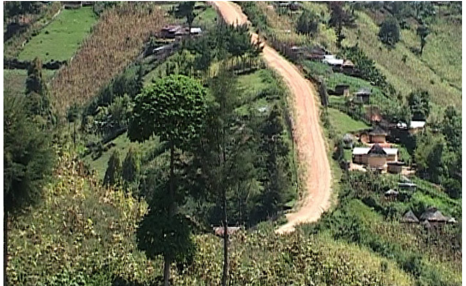
The 6km Maina – Chemworor road in Tot Sub-County built through public participation
